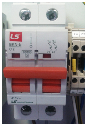
Figure 10: Two-pole circuit breaker for the auxiliary power circuit.
